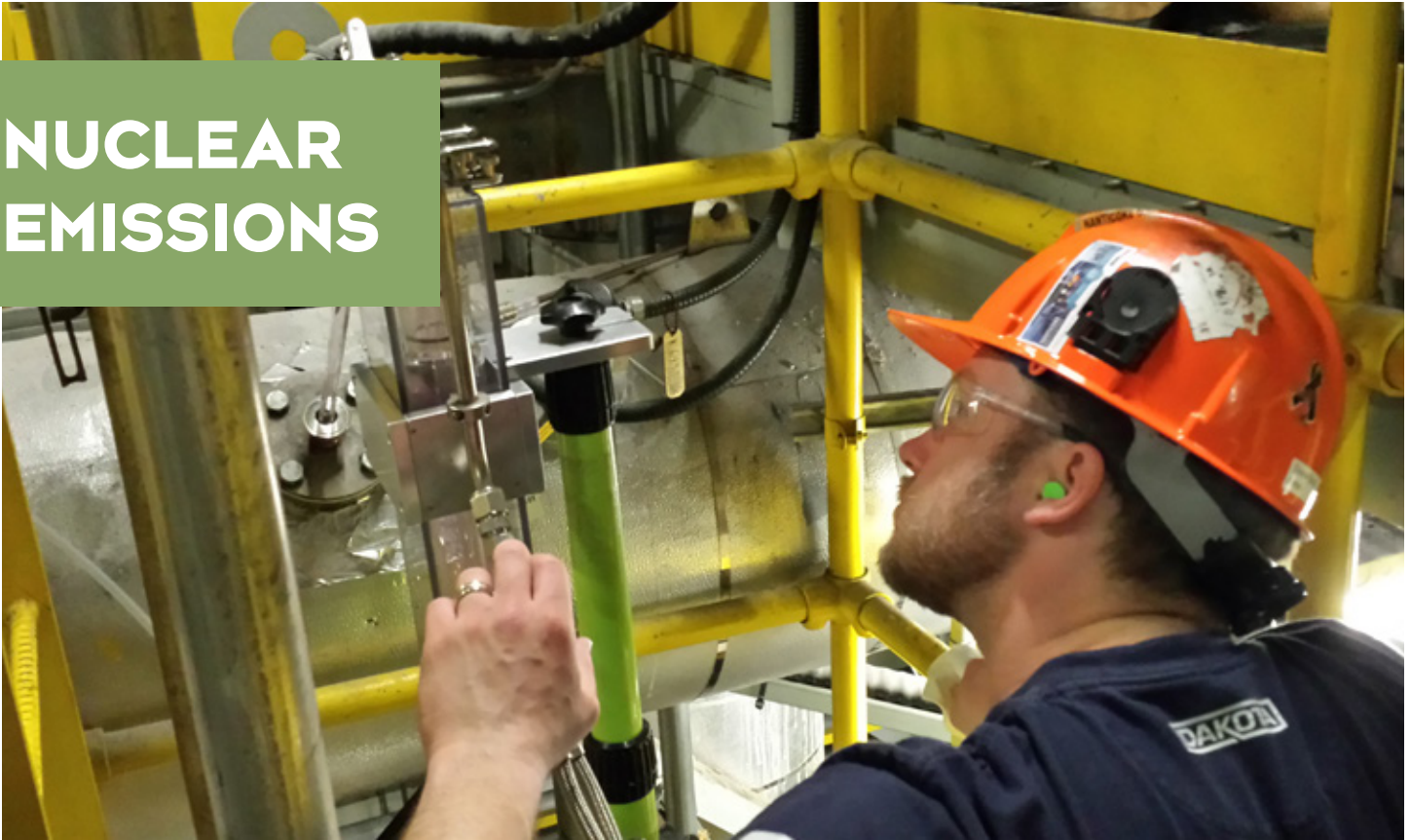
Setting up an emissions monitoring system test.
