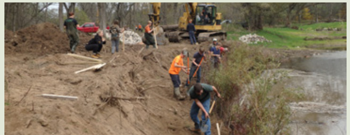
Students working to prevent stream bank erosion along Catfish Creek.
