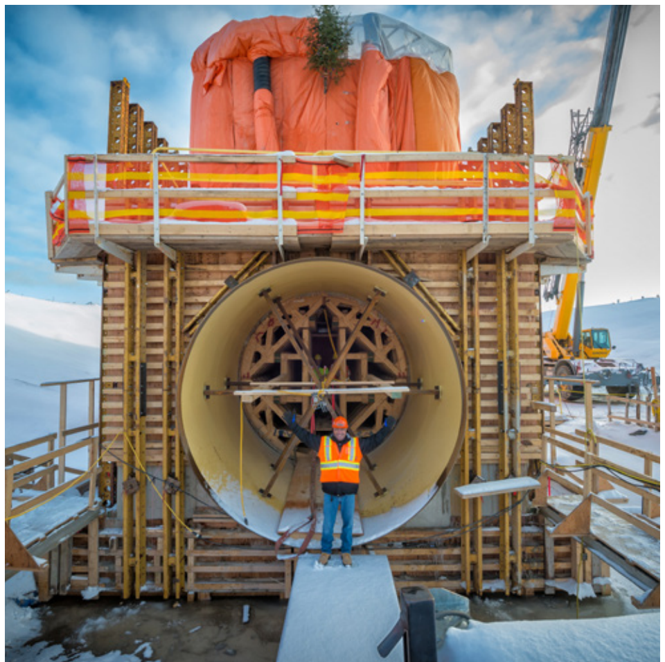
Construction of the Peter Sutherland Sr. GS.
